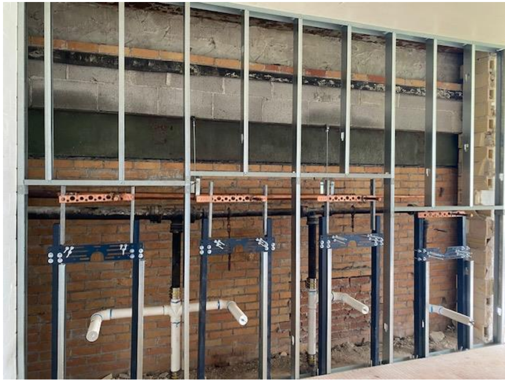
Chase Wall Plumbing Complete
