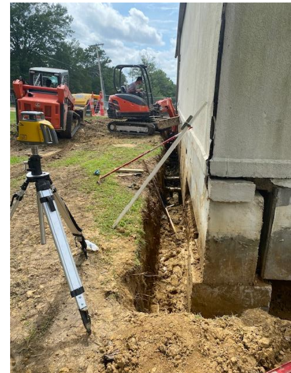
Perimeter Excavation
